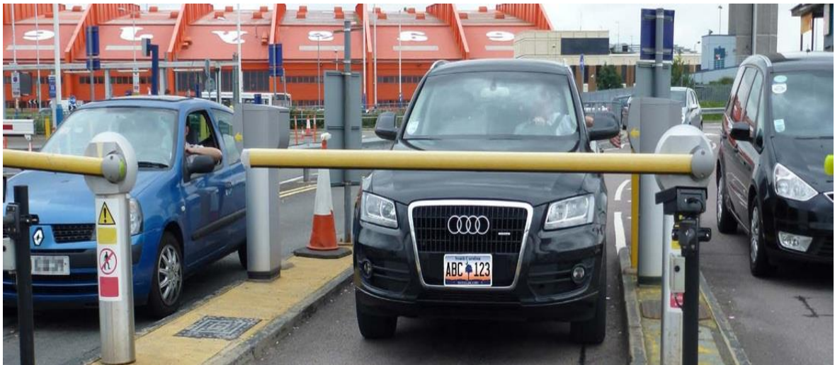
Figure 4.1: Typical ANPR and Barrier Access Control
